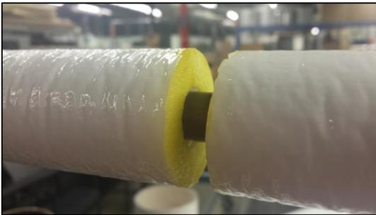
Figure 5: Adhesive applied to butt ends of insulation
