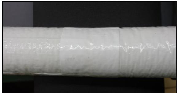
Figure 6: Sealed Butt joint with additional butt joint tape
